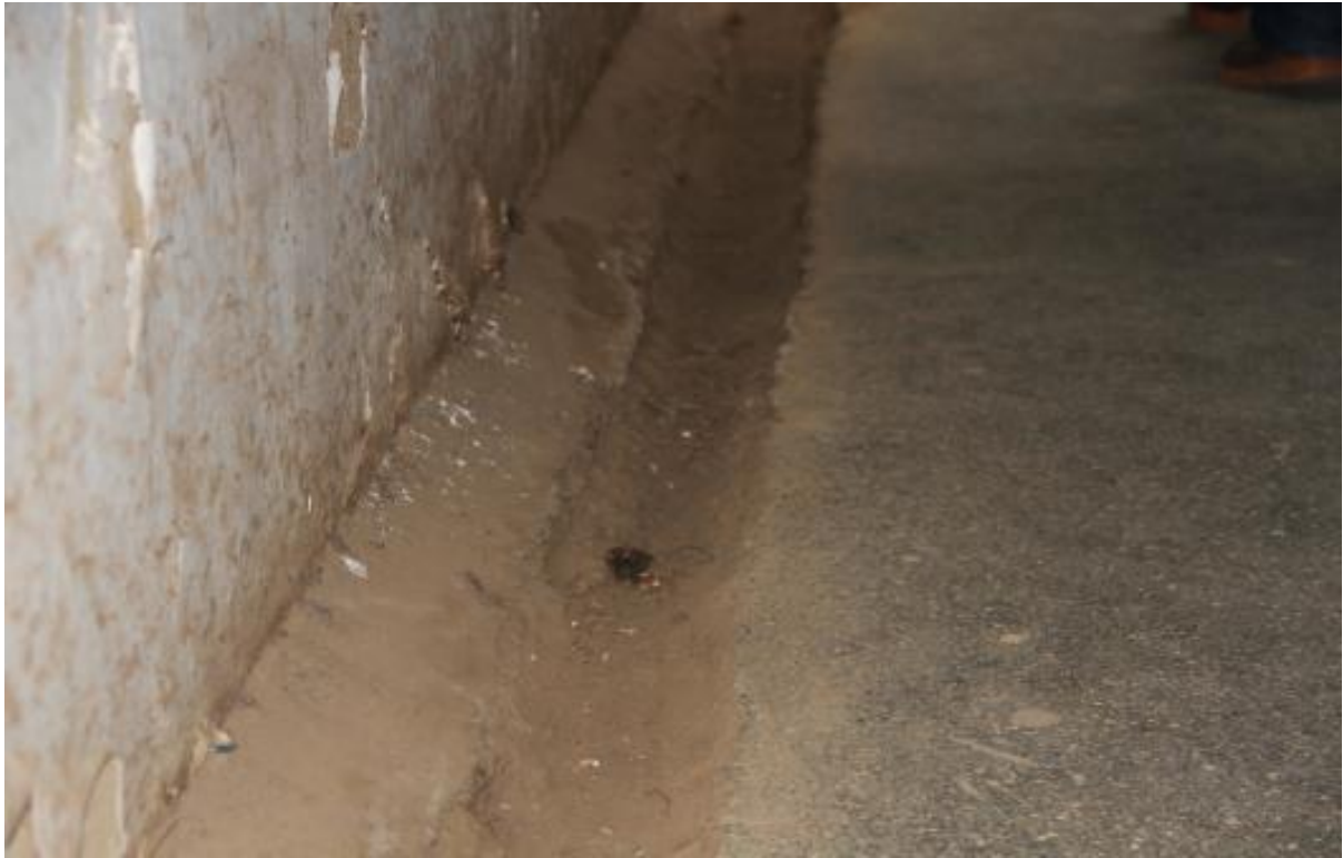
Plate 4-14: Longitudinal Drainage Pan within the Tunnel (Author, 2016)
