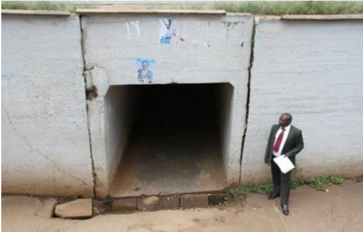
Plate 4-5: Lateral Displacements of the Retaining Wall Panels (Author, 2016)
