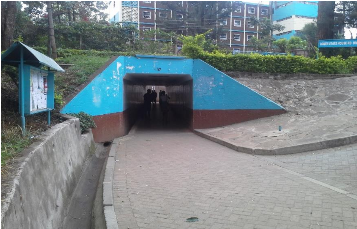
Plate 5-6: Illustration of Underpass Drainage Pan (Author, 2016)
