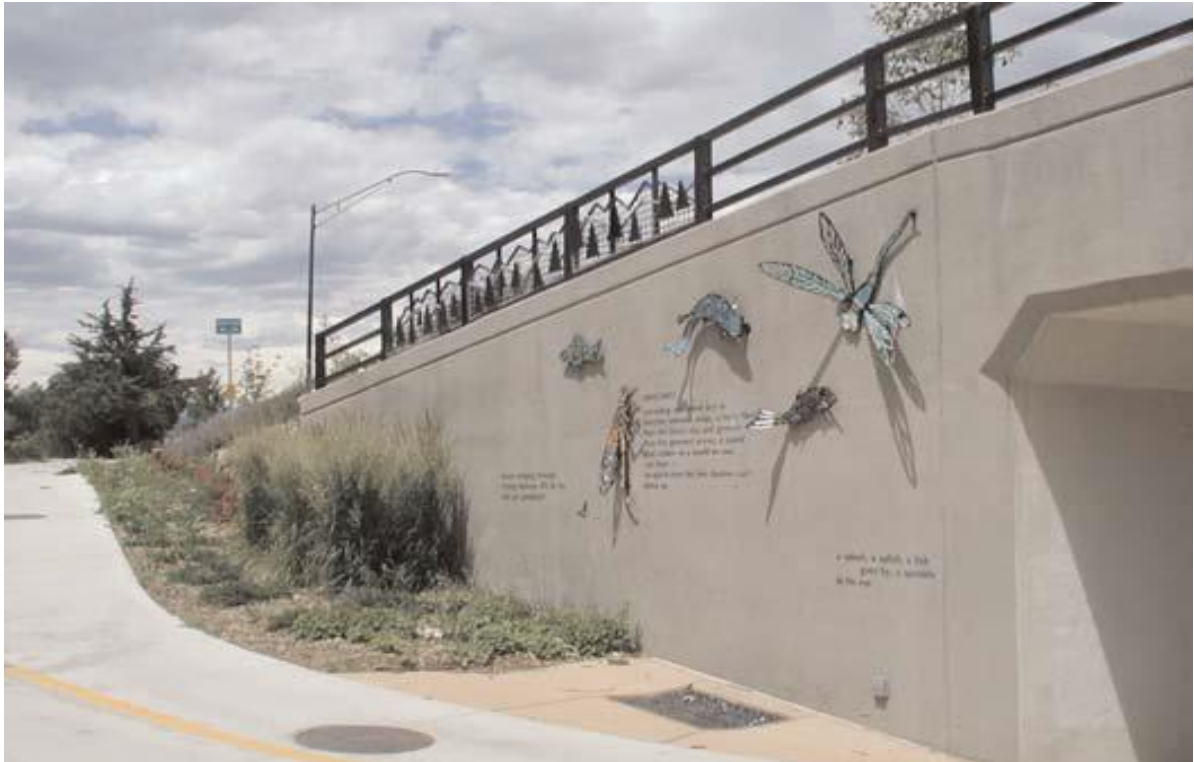
Plate 5-4: Illustration of External Artwork on the Retaining Wall (City of Fort Collins , 2001)
