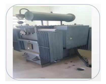
Figure 1.2: 630KVA Transformer serving Equatorial Fidelity Centre
