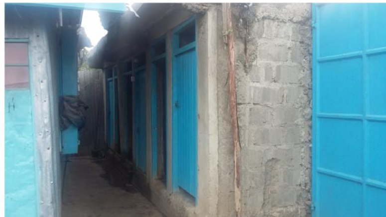
Plate 5-1: Washrooms within the Building Line Space
