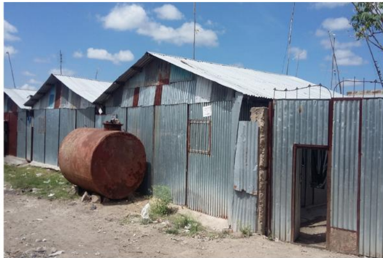
Plate 5-4: Connected Structures Source: Fieldwork, 2016
