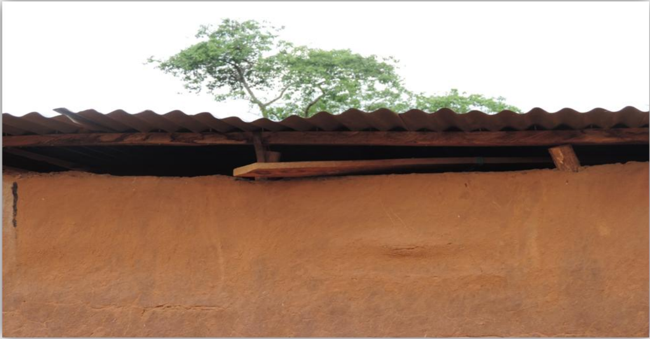
Picture 4. 5: Corrugated iron roof and mud wall house with wide eaves
