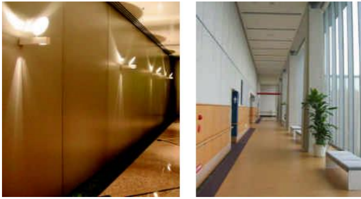
Figure 2. 4: Lighting walkways and the placement positions of light fittings to avoid barriers
