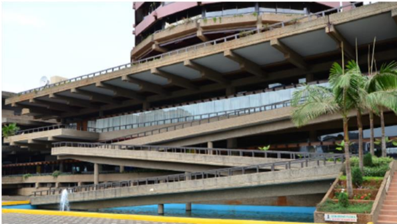
Figure 2. 1: Antrance with accessible stairs and ramps at KICC building Nairobi, Kenya
