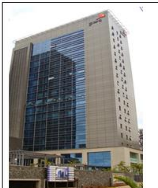
Plate 4.4: Delta tower along Waiyaki way in Westlands, Nairobi Source: Research, (2015)
