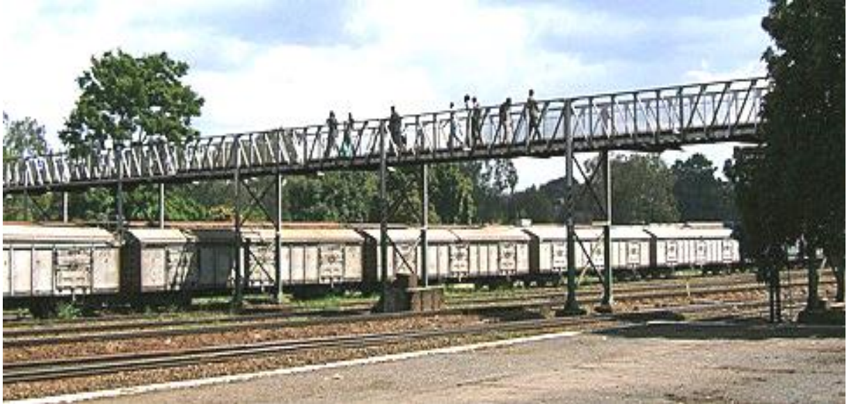
Figure 2.1: Footbridge as Viewed from the Railway Station Platform
