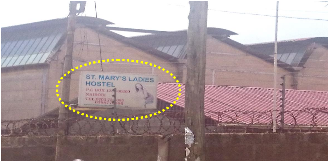
Figure 2.12: Conversion of Railway Workshops to Student Hostels
