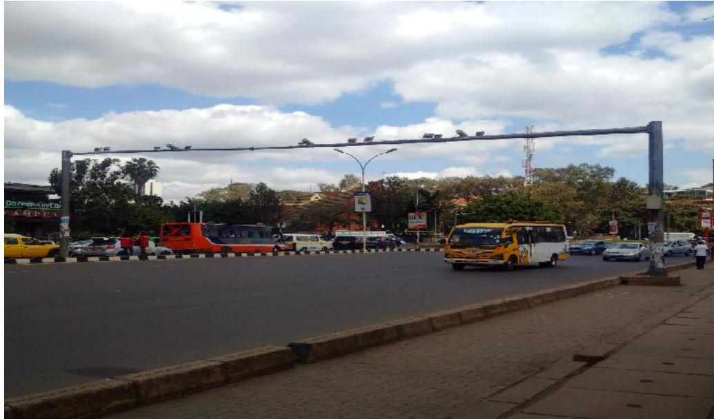
Figure 1: CCTV Cameras along University way (field data)
