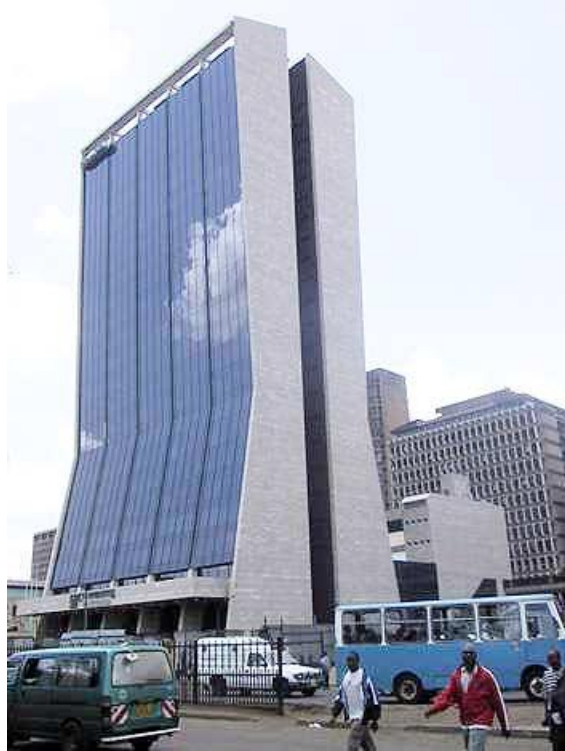
Figure 5: Refurbished Co-operative house after US embassy terror attack. The structure never collapsed due to its structural resilience
