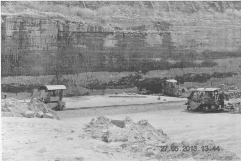
Plate 2.2: Stone cutter machines at work in a quarry in Juja
