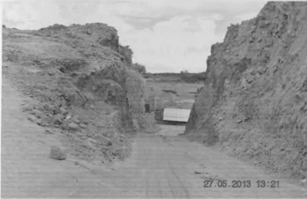
Plate 2.4: Loose rocks at an entrance to a quarry site
