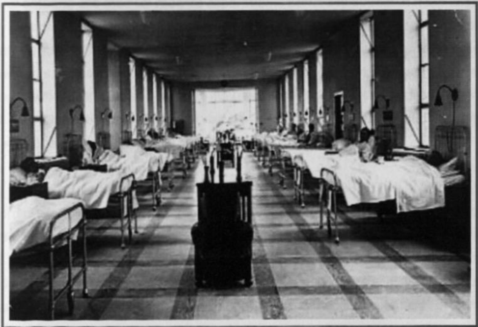
Figure 3.1: An interior view of a typical "Nightingale" ward
