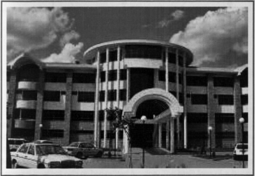
Figure 3.7 Karen hospital, an example of a modern hospital in Nairobi, .
