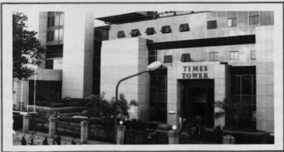
Figure 2.12: Times Towers, Headquarters of The Kenya Revenue Authority (KRA). An example of a district
