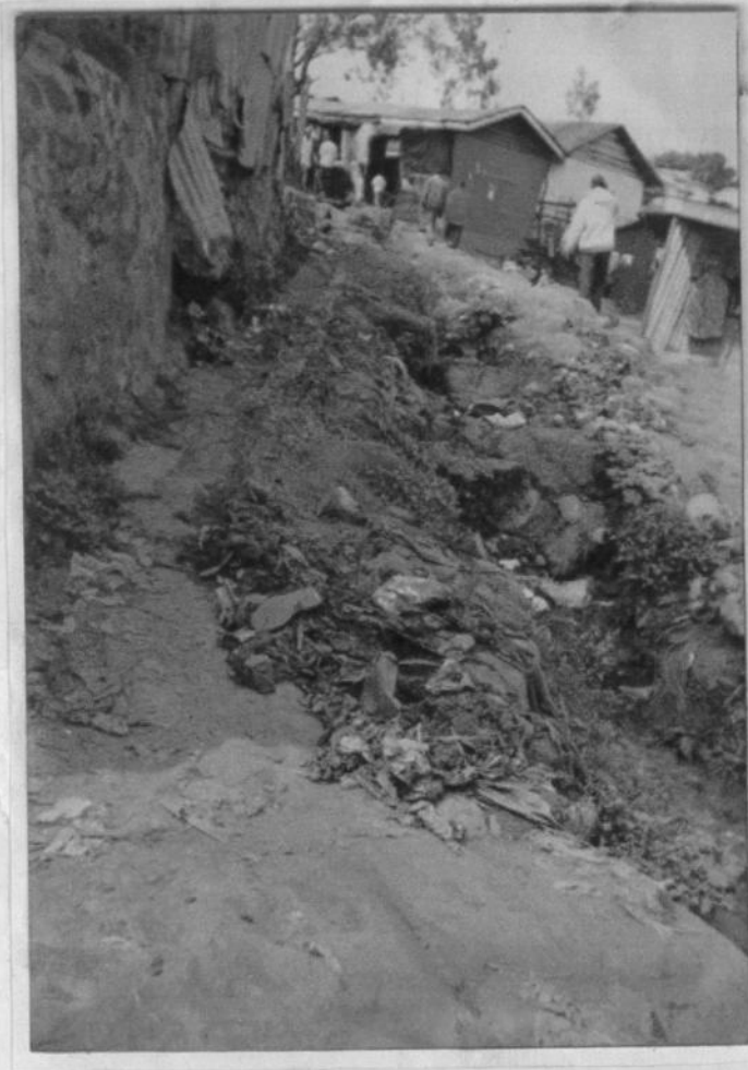
Plate 3: Dirty Drainage: After an Attempted Clean-Up in Kibera
