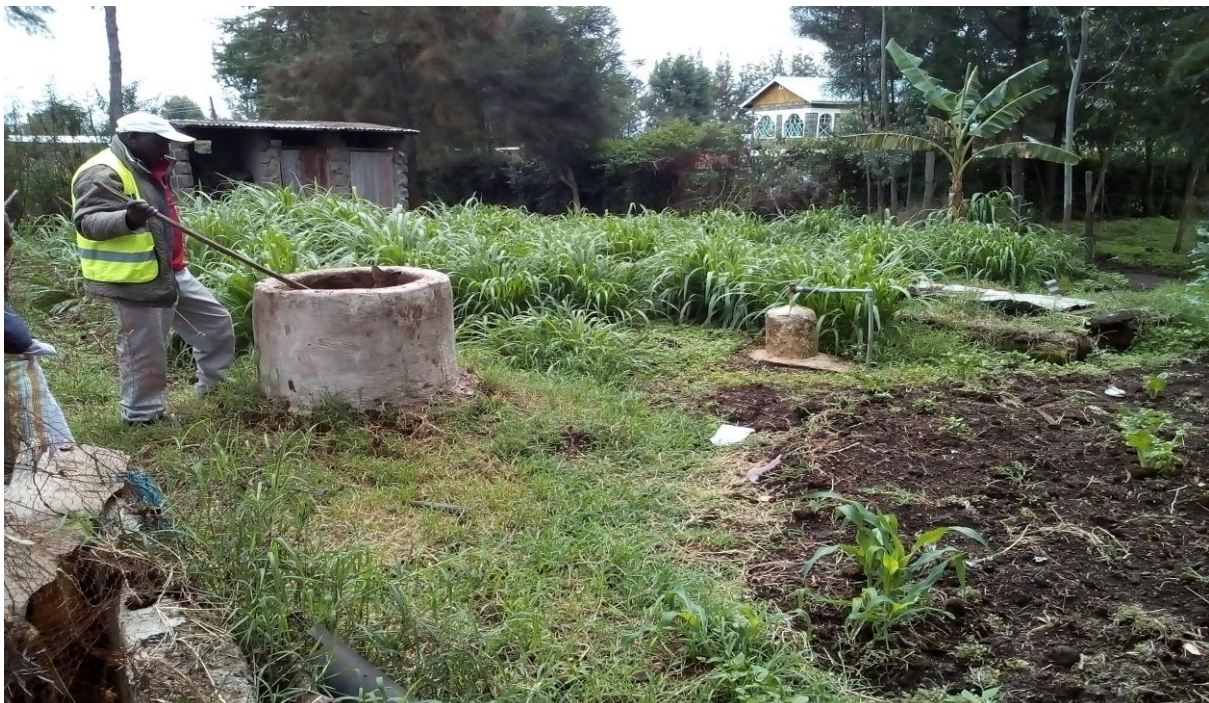
Plate 2: Biogas production system
