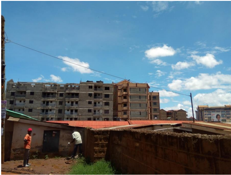
a) On-going constructions in Ruaka Town
