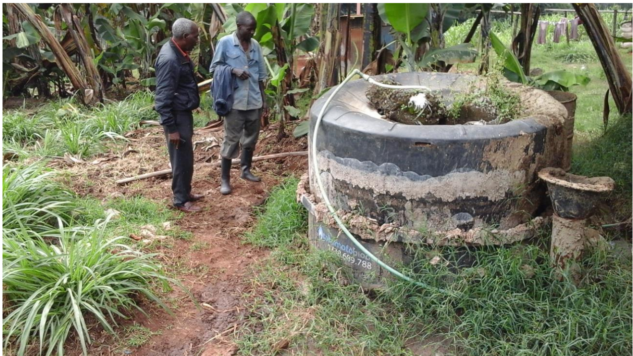
Figure 4: A floating drum bio-digester made of polyethylene in Githunguri sub-county
