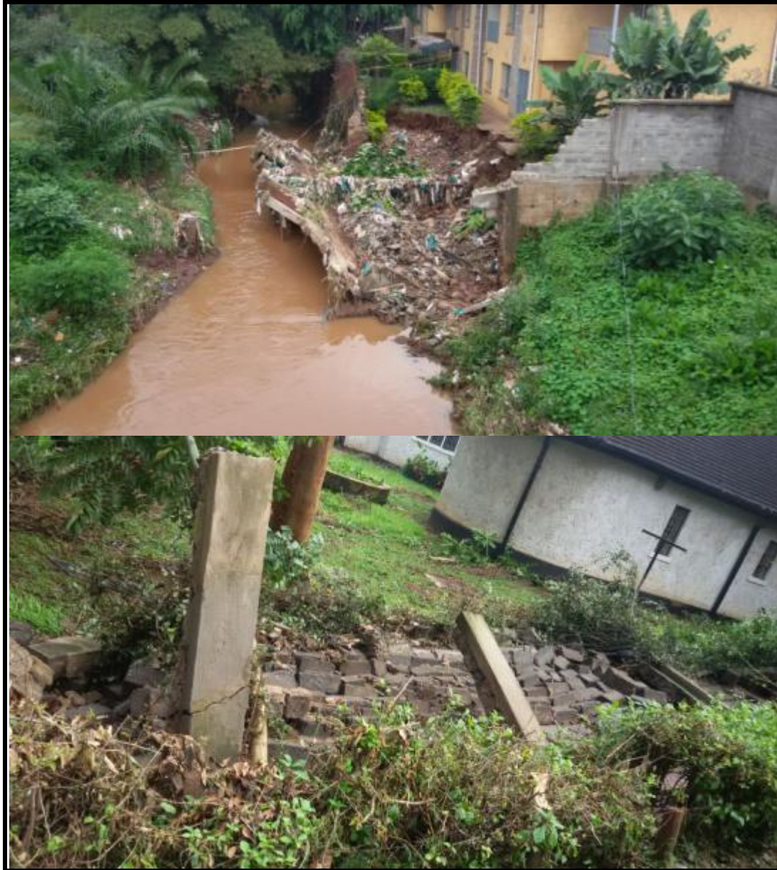
Plate 4-10: Demolished walls in Kileleshwa Estate by floods
