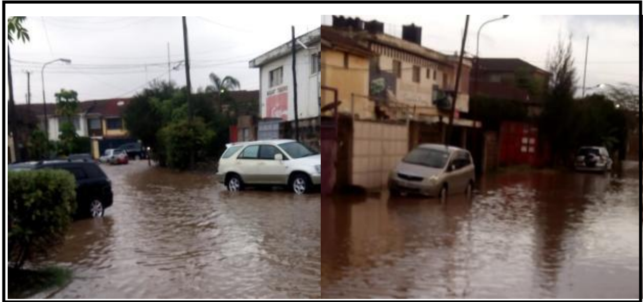
Plate 4-8: Flooded sections of South Cs Mugoya estate
