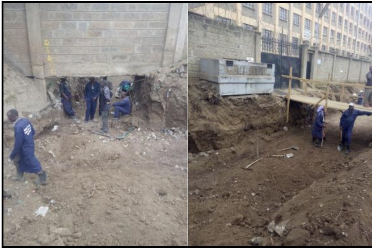
Plate 4-13: Drainage systems being cleared by County government of Nairobi
