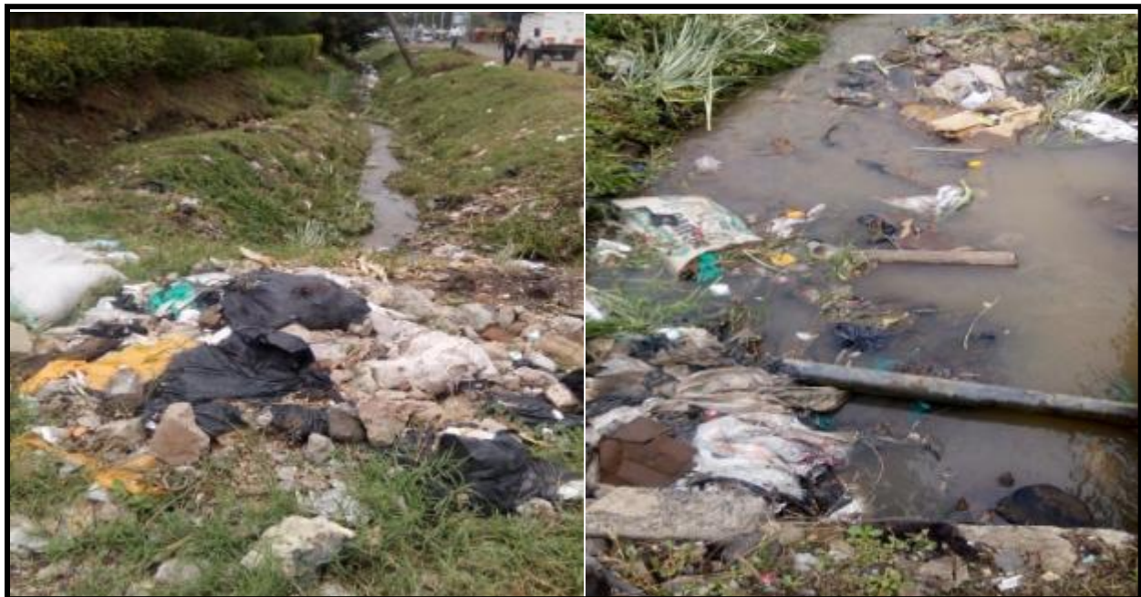
Plate 4-4: waste poorly disposed off on the drainage system
