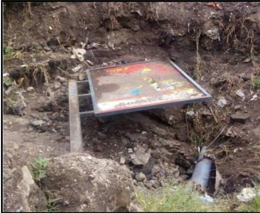
Plate 4-9: Sign board fell by the heavy flood rains at South C shopping Centre
