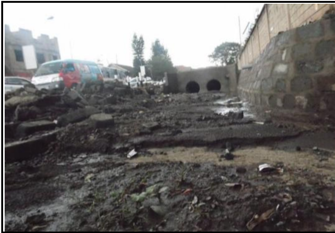
Plate 4-12: Culvert and trench constructed by County government of Nairobi
