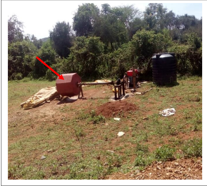
Plate 4.2: Unguarded crusher at mine site 3 Source: Research Field Visits, (2018).
