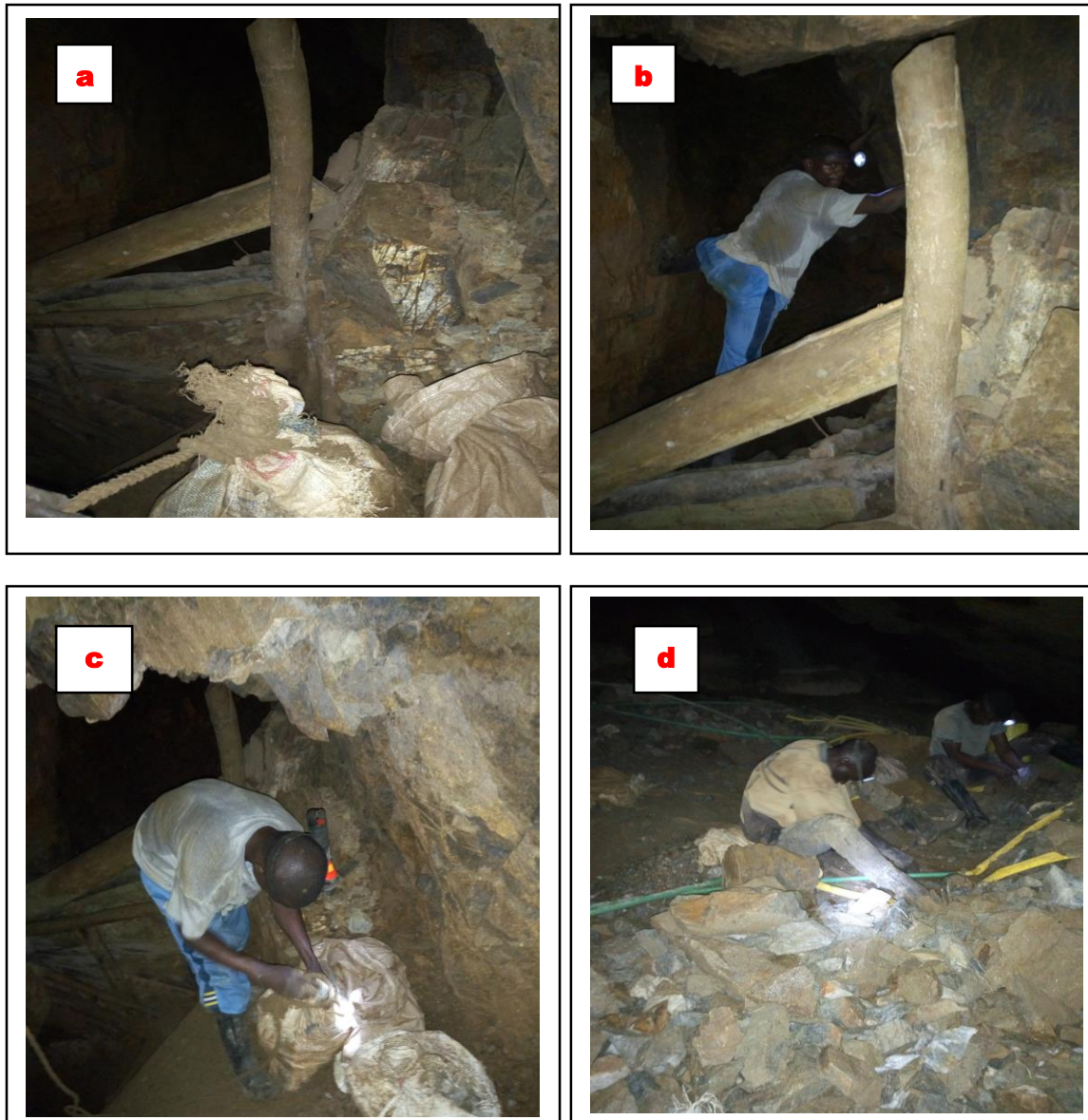
Plate 4.1: Underground workings; (a) deteriorated timber support, (b) inadequately supported stopes, (c) a miner lifting heavy load while bending over hanging rocks & (d) miners sitting in an awkward position while excavating the rocks.
