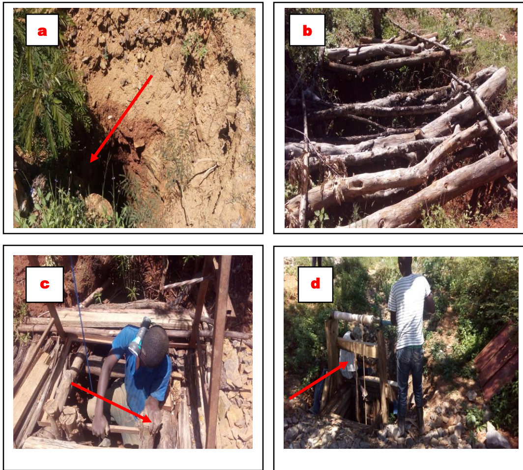
Plate 4.7: Deplorable safety conditions & Risky behaviours (a) Uncovered shaft, (b) Deteriorated timber support (c) A miner holding a timber with bare hand & (d) A miner hanging on a shaft while removing ore.
