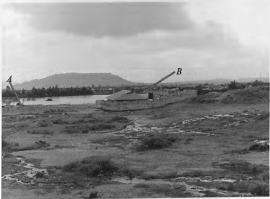
Figure 4.24 : Encroachment on a Site Meant to be a Dam. (The only dam in Maai Mahiu Division) Nb: the Waterways Leading to the Dam.
