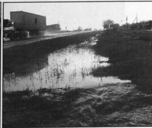
Figure 5.3: A section of the Maai Mahiu-Naivasha Highway
