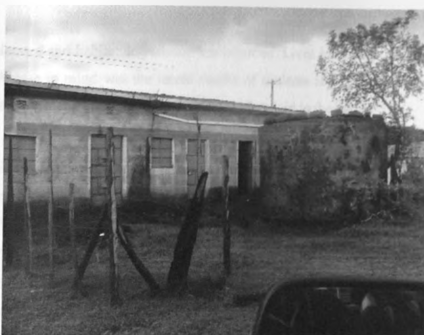
Figure 5.1: Homestead with a Water catchment System - Longonot Township
