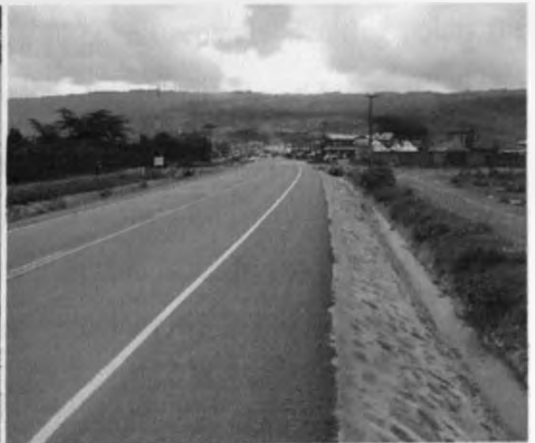
Figure 5.9: Storm drains on part of the Maai Mahiu – Narok Road
