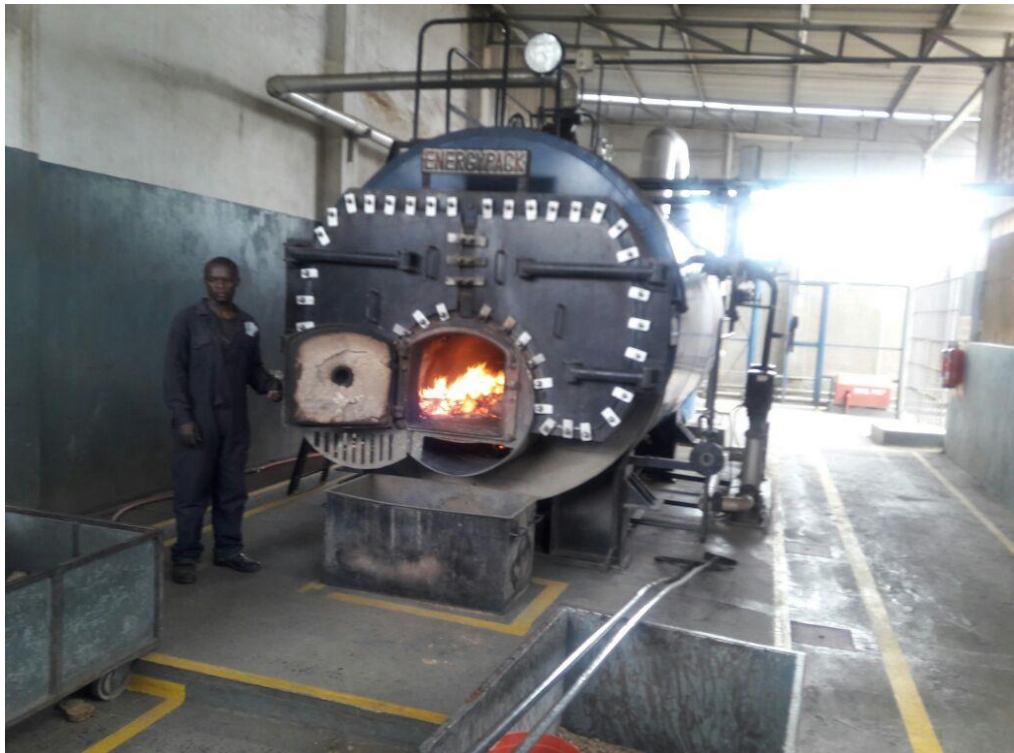
Plate 2: A Briquette fired boiler in operation at Meru Dairy Co-operative Ltd in Meru County
