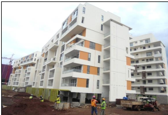
Garden City Apartments – Thika Road (Source: Field Survey, 2017)
