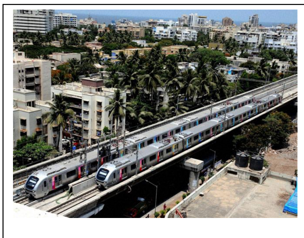
Figure 2-3 Metro trains running on rail track in Mumbai
