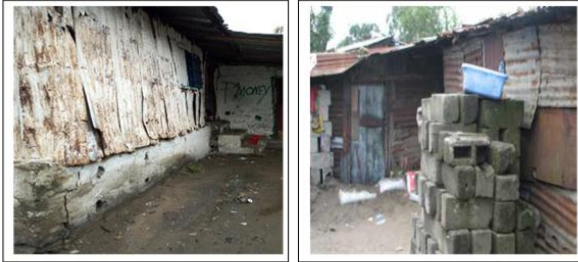
Plate 4.2: Housing Condition: Houses built with old aluminium sheets and without proper ventilation
