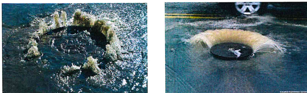
Picture 1a and 1b: Sewer surcharges on the streets after the conduit capacity is overwhelmed.
