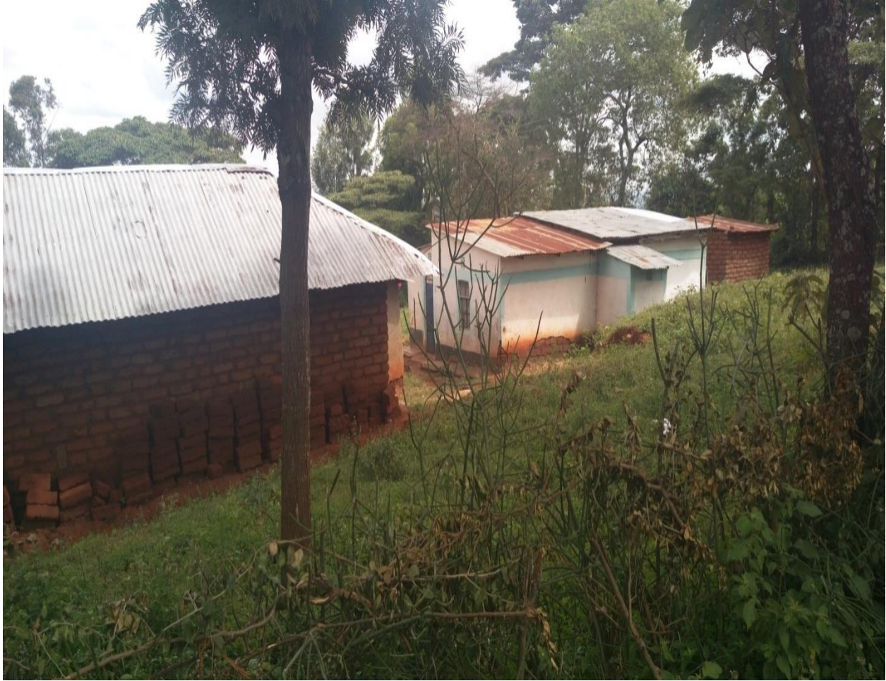
Plate 8: A house made of brick walls with a roof made of corrugated iron sheets
