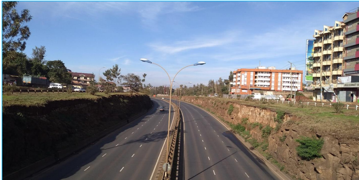
Figure 4-3; Curve at Juja Interchange
