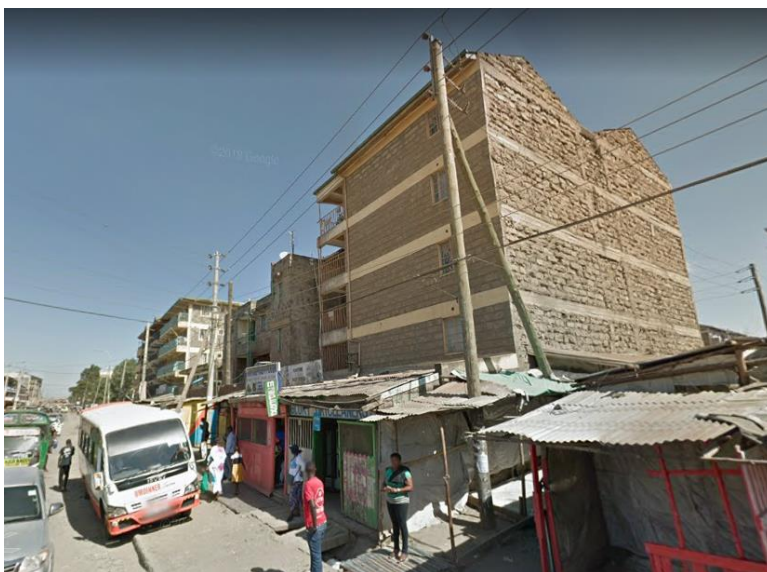
Figure 4.2: Informal Buildings along Way Leaves and Pedestrian Walkways
