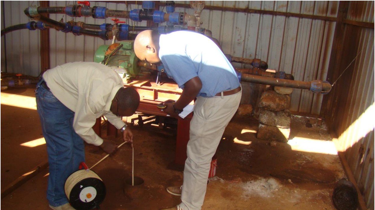
Figure 3.4: Taking borehole water rest level measurements using a dipper.
