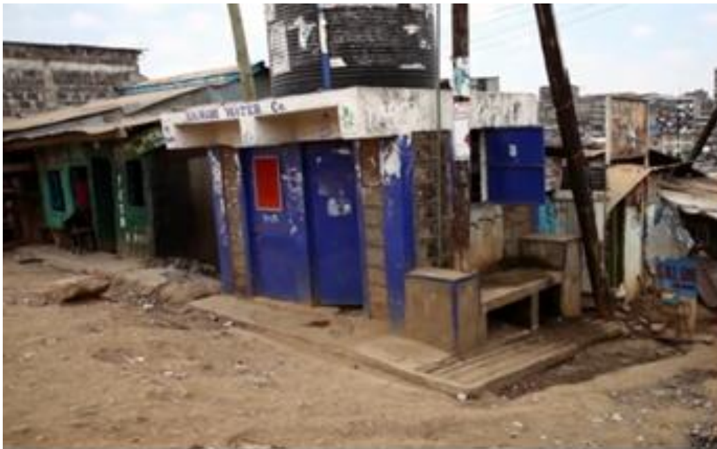
Photo 1: Water kiosk installed during the partnership
