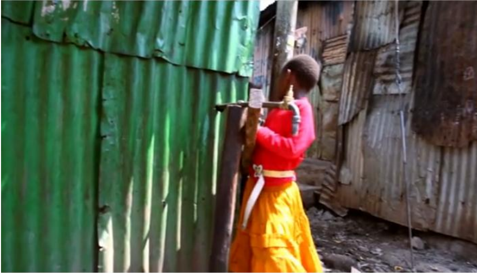
Photo 2: A yard tap installed within the household premises (plot)
