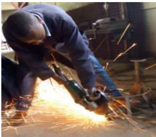
Plate 8-6(a): Plenum system fabrication
