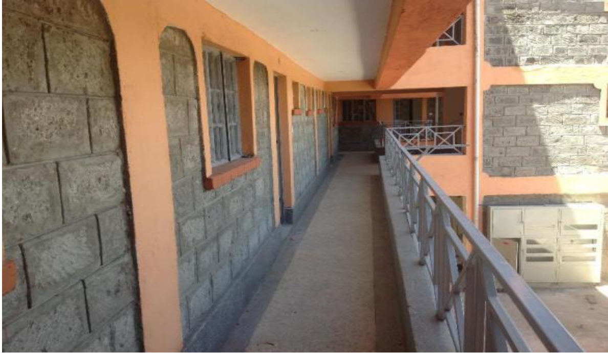
Figure 4. 4 : Middle Income Residential buildings; Imara Diama and Pipeline Estate, N. East.
