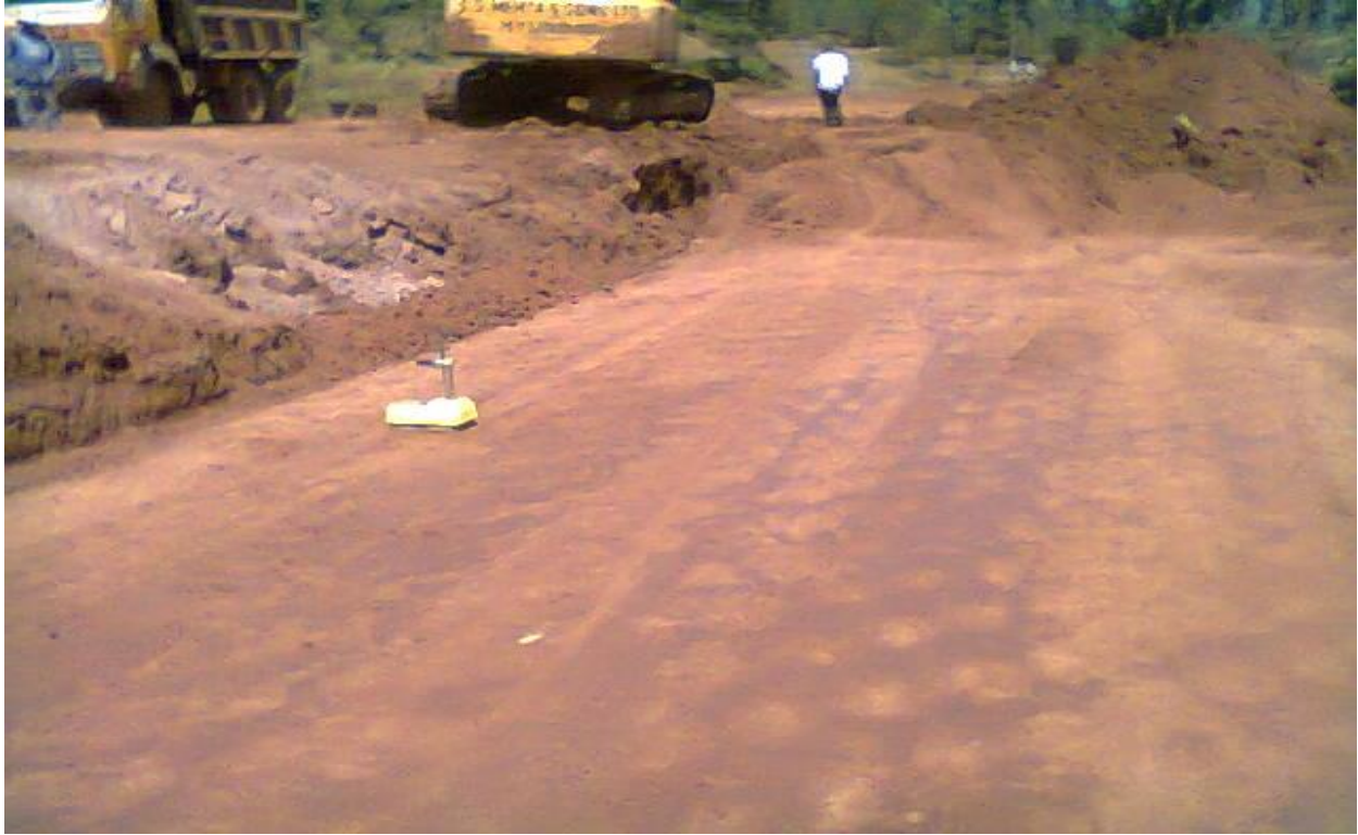
Figure 1-2: Use of nuclear gauge at a construction site- workers keep distance during density tests
