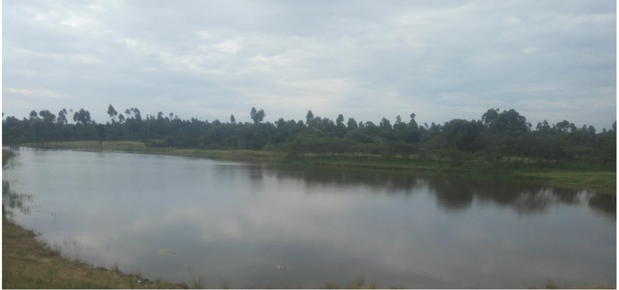
Figure 3.8 Kaposur Earth Dam
