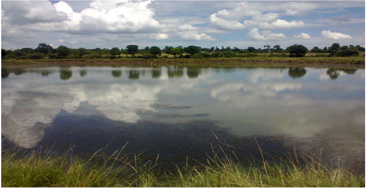
Figure 3.4 Birir Earth Dam
