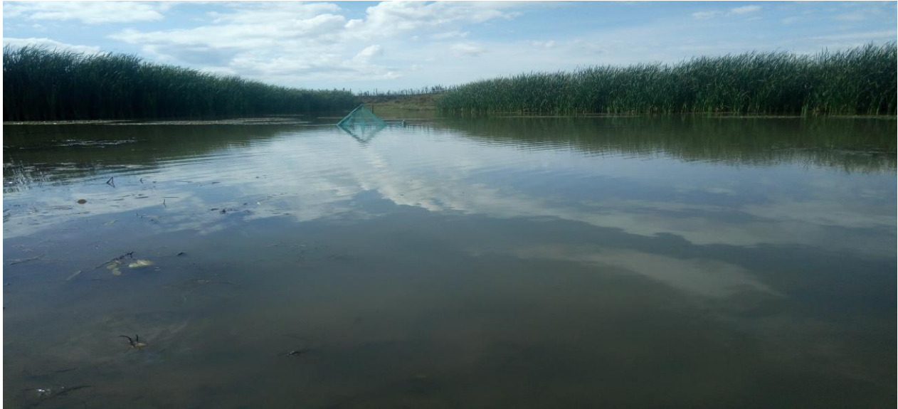
Figure 3.7 Sogororbei Earth Dam
