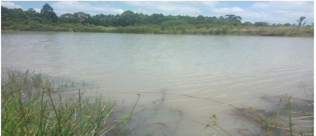
Figure 3.5 Cheboloigo Earth Dam
