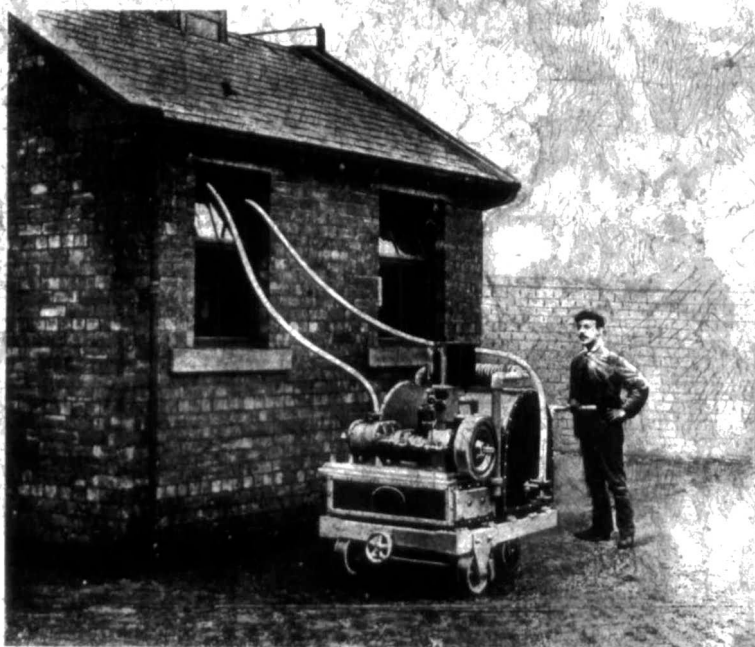
INFECTED PREMISES UNDERGOING FUMIGATION BY PORTABLE MACHINE, TYPE "H."
