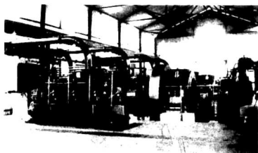
KIMINGSI - POWER HOUSE INTERIOR.
