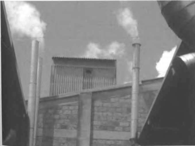
Photograph 4.12 Flash steam and hot vapor from drier exhaust
