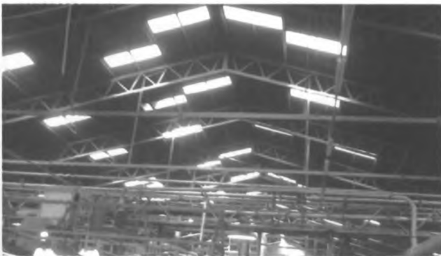
Photograph 4.14 Roof sky light showing ceiling lights off during the day
