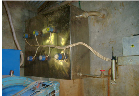
Fig. 6 The six 3kW each Dumpers (Ballast)
