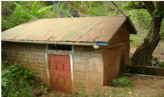
Fig. 3 The Power House
