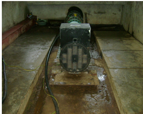
Fig. 30 Turbine and Generator mounting
