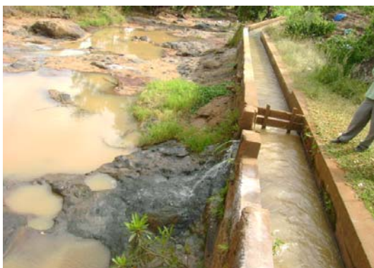
Fig. 9 Tungu River – all water diverted to the channel
