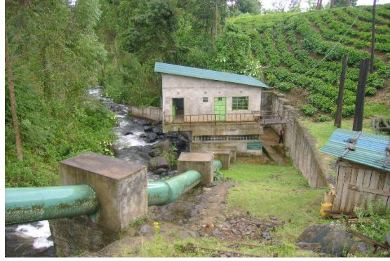
Fig. 22 the power house
