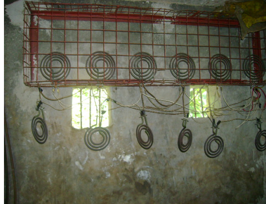
Fig. 39 Electric Coils as Power Dumpers
