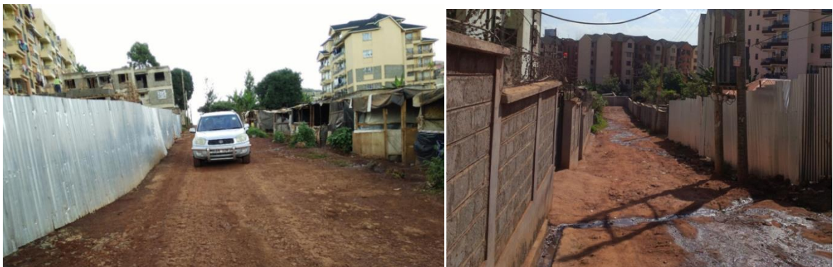
Plate 5-9: Narrow Roads That Lack NMT/Drainage Wayleaves along Access Roads.
