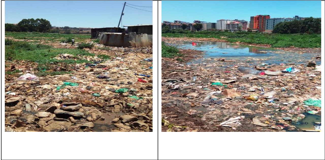
Plate 4. 2: Pictures showing plastic waste dumped inside the dam
