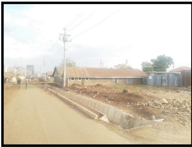
Plate 1: Improved road surface and storm water drain (Source: Field study)
