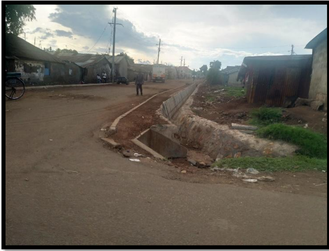
Plate 6: Road surface and pedestrian walkway. (Source. Field survey)
