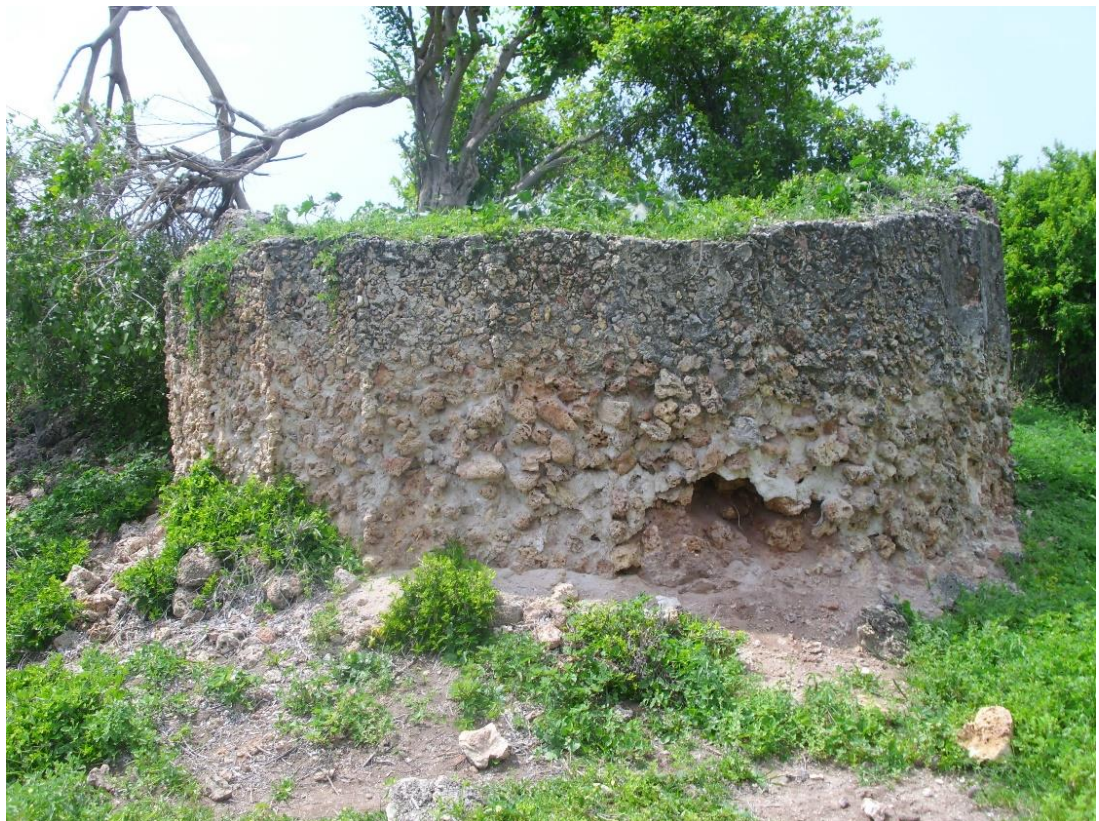
Plate 4. 1: A section of the bastion along the southern town wall.
