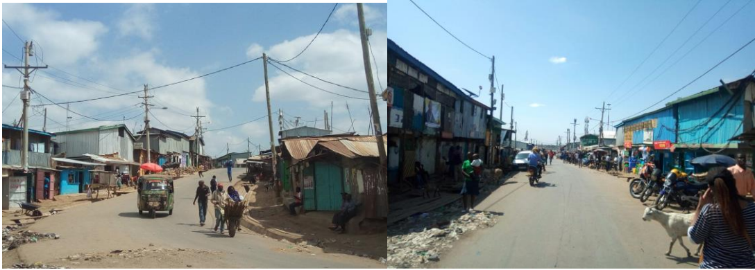
Plate 10: Electricity Network Along the Main Road
