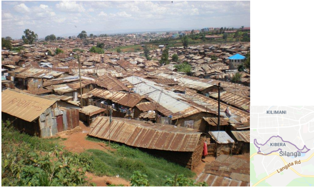
Plate 4: Silanga Village Current Power Connection Status
