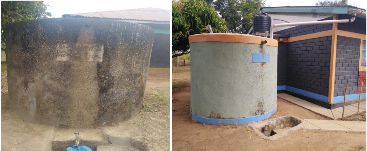
Plate 8: KWG self-sponsored water harvesting project – cement water tanks
