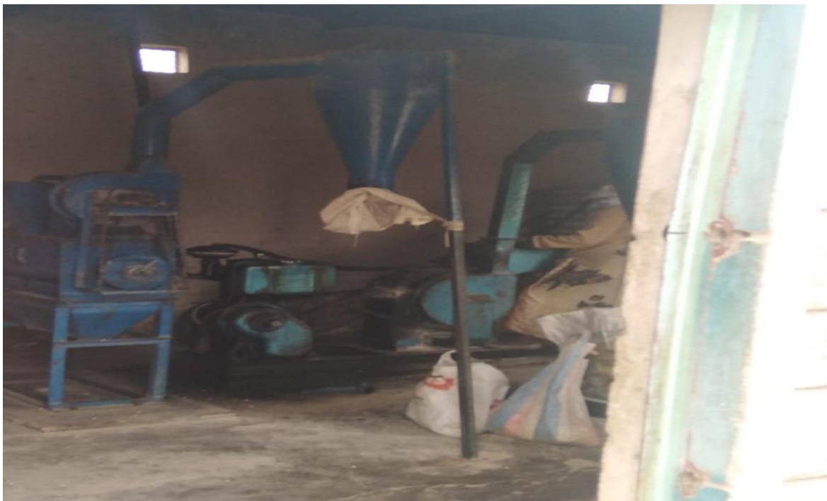
Plate 7: KWG Posho Mill Project
