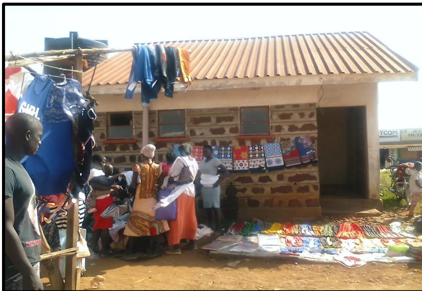
Figure 8: Public Toilets in Funyula market
