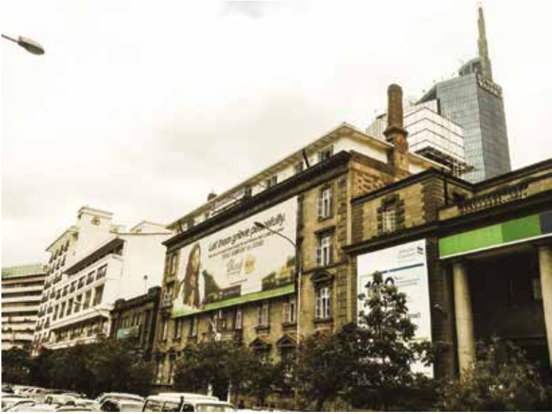
Figure 5.2 Symmetry, use of pediments, rustication, quoining and cornice on Panafrican House ( http://nairobians.net/ , accessed February 2016)
