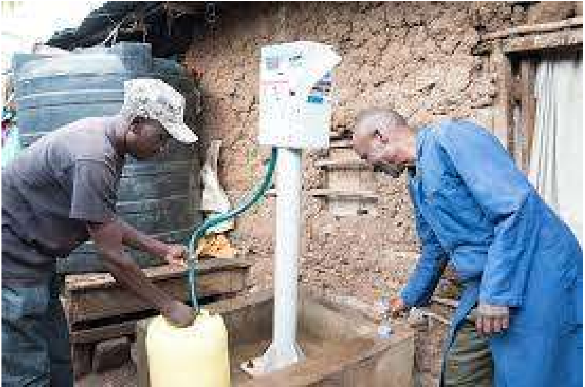
Communal prepaid meter in Nakuru ( Source: Author)
