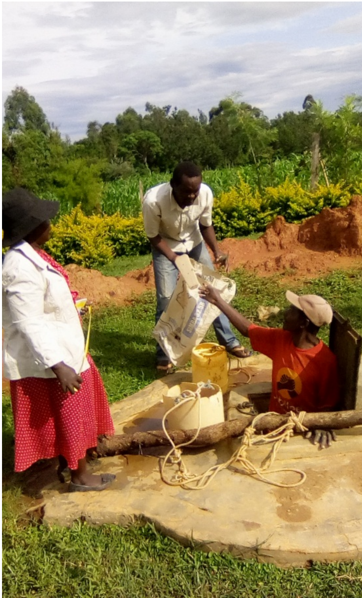
Photo 1: The artisans rehabilitating a shallow well
