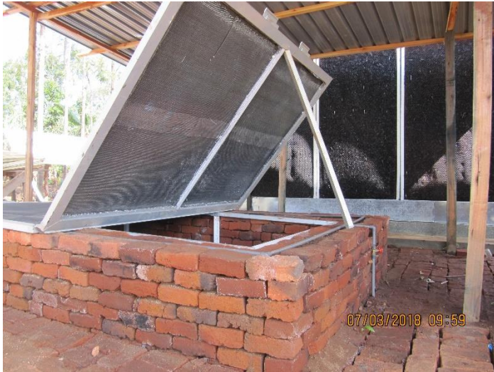
Figure 4.1: Side-view of the Zero Energy Brick Cooler (Source: Karurumo Smallholder aggregation and processing center, Embu County)
