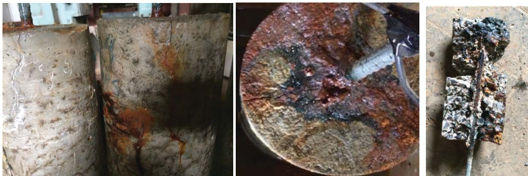
Figure 3.4 Images of corrosion samples after corrosion.
