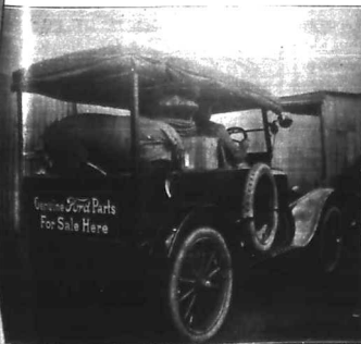
Ford Service Car proceeding to the Lake River Station.
