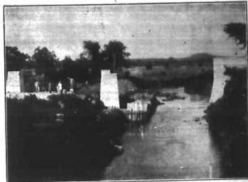
Bridge construction on the new Kitale Branch Railway Line.
