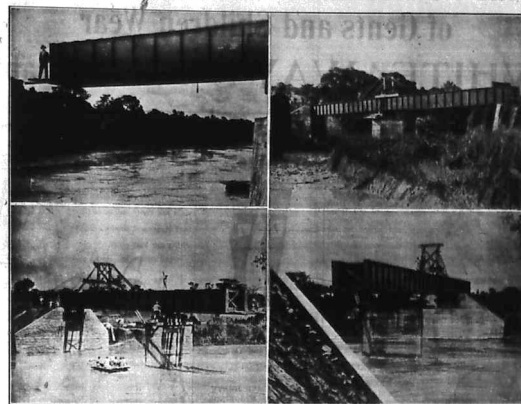
Railway extension into Uganda: Bridging the Nusia River, 25 miles from Turko. The photographs show a novel method of launching employed by Mr. H. G. Dempster, the Resident Engineer. The ends of the two girders are suspended by means of levers passing over the trestles. The bridge has a span of 130 feet. The railway is being built departmentally. Photo: W. H. Stevens.
