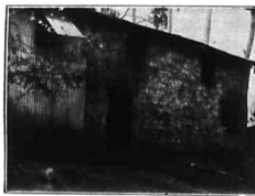
Tenement dwellings in Nairobi rented by Africans. The building consists of a number of rooms each rented at about Shs. 10 per month.
