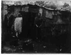
African dwelling constructed of scrap material.
